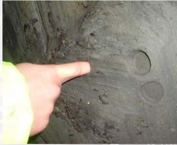
Unmixed Material Adjacent to Columns
