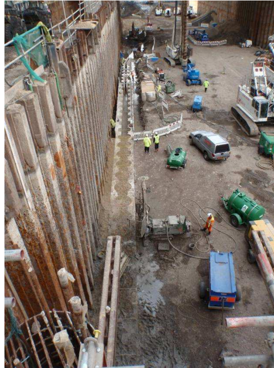
Guide wall installation
