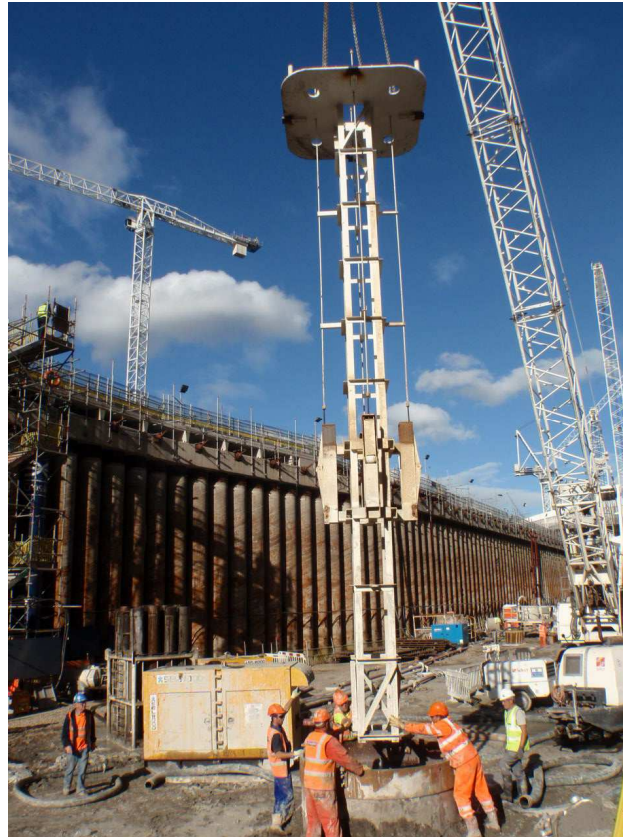
Plunge column guide frame installation
