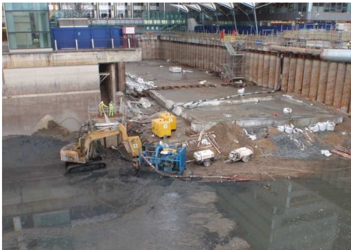
Dock silt removal – wash and pump
