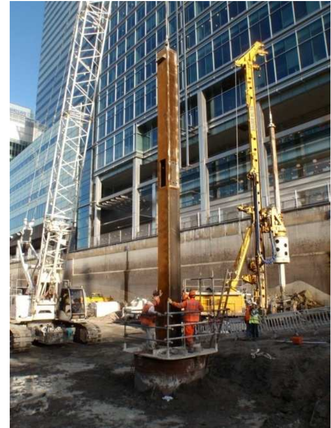
Plunge column installation (18m long, upto 27t)
