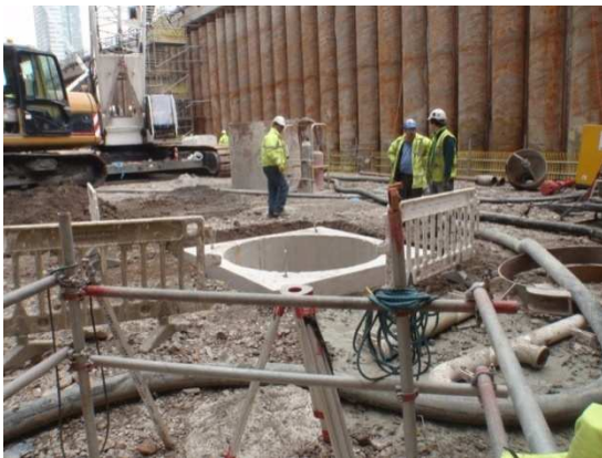
Precast guide hole for 2.1m pile
