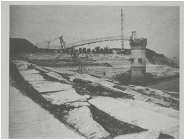
FIG. III - 18 SLIDE DAMAGE NEAR WEST ABUTMENT - LOWER SAN FERNANDO DAM
