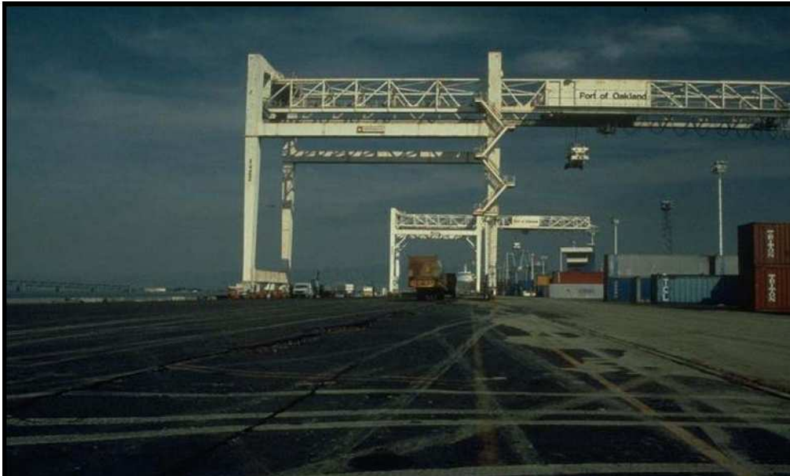
1989 Loma Prieta Earthquake – Port of Oakland 7th Street Marine Terminal Source – R. Kayen, U.S. Geological Survey and Loma Prieta Collection, Earthquake Engineering Research Center, University of California, Berkeley
