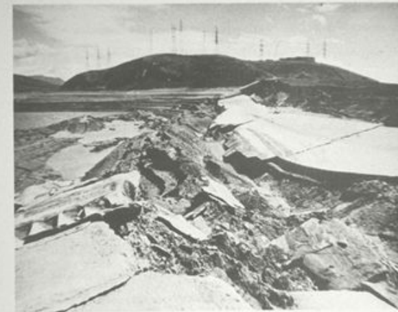
FIG. III - 22 SLIDE DEBRIS - LOWER SAN FERNANDO DAM
