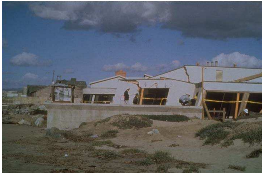
1989 Loma Prieta Earthquake – Moss Landing Marine Laboratories Showing structure “stretched” more than 5 feet due to lateral spreading Source – L. Harder, Loma Prieta Collection, Earthquake Engineering Research Center, University of California, Berkeley
