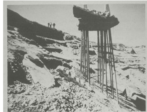
FIG. III - 21 PILE-SUPPORTED FOOTING FOR BRIDGE TO CENTRAL OUTLET TOWER - LOWER SAN FERNANDO DAM
