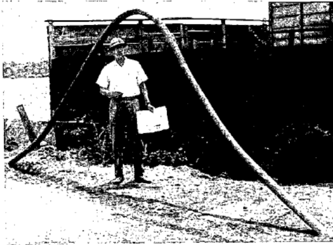
Photo 31 Buckling of a Buried Gas Pipe
