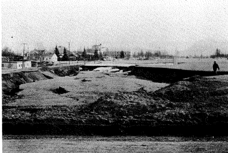
Fig.33-GRABEN BEHIND 'L-STREET' SLIDE AREA, ANCHORAGE (1964).
