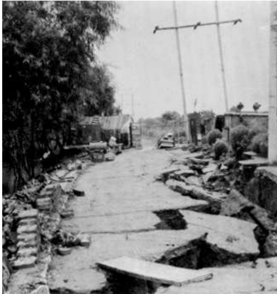
Figure 23. Damage to road near Loting Hsien. Slumping, lurching and settlement of soft soils caused extensive damage to highways in the Tangshan region.
