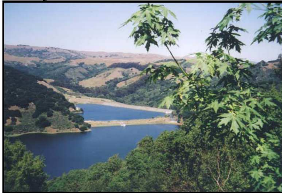
Upper San Leandro Reservoir showing original hydraulic fill dam and newer replacement dam Source – J. Perkins, ABAG
