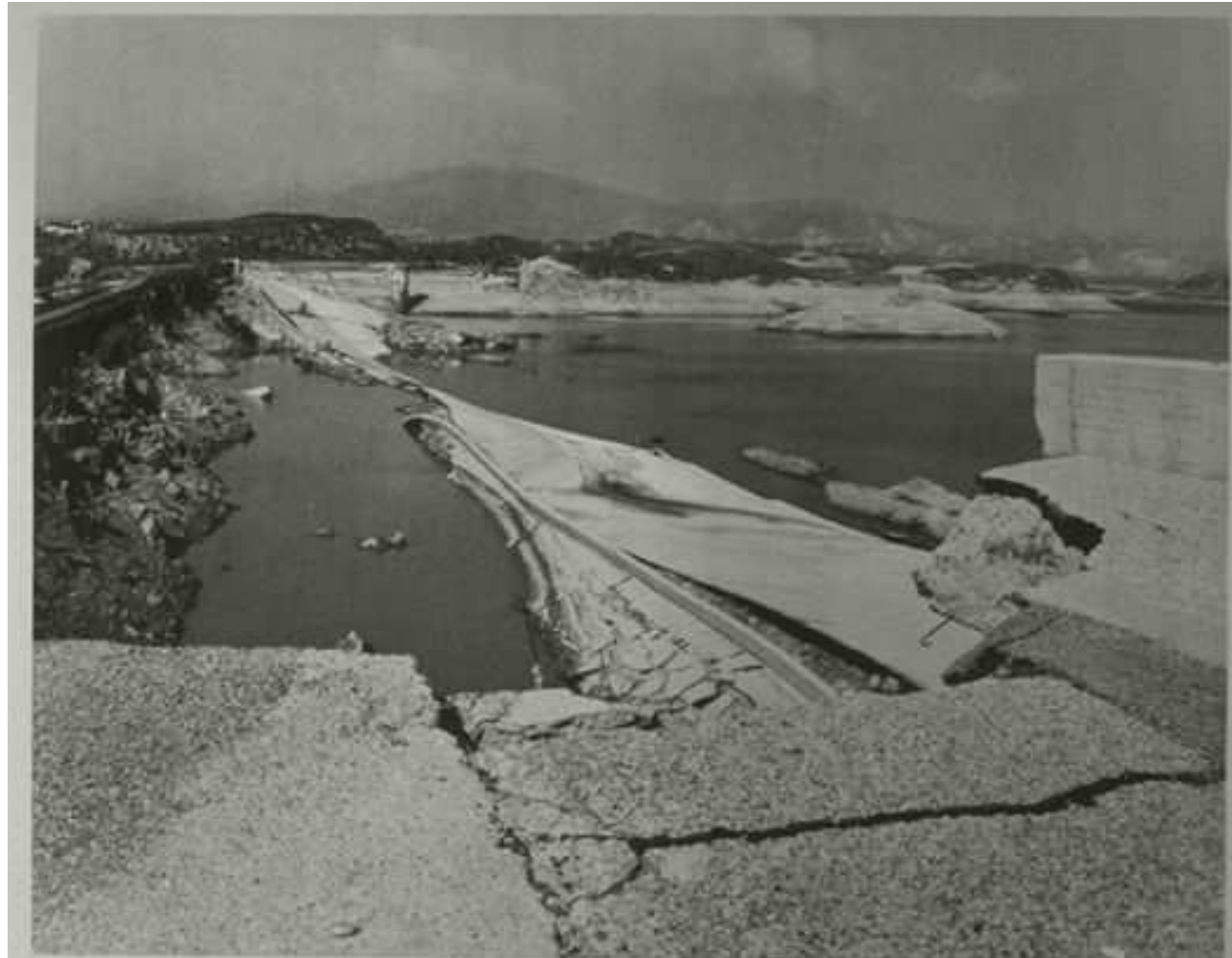
FIG. III-17 SLIDE DAMAGE TO LOWER SAN FERNANDO DAM. (Photograph by Department of Water Resources, Feb. 22, 1971)
