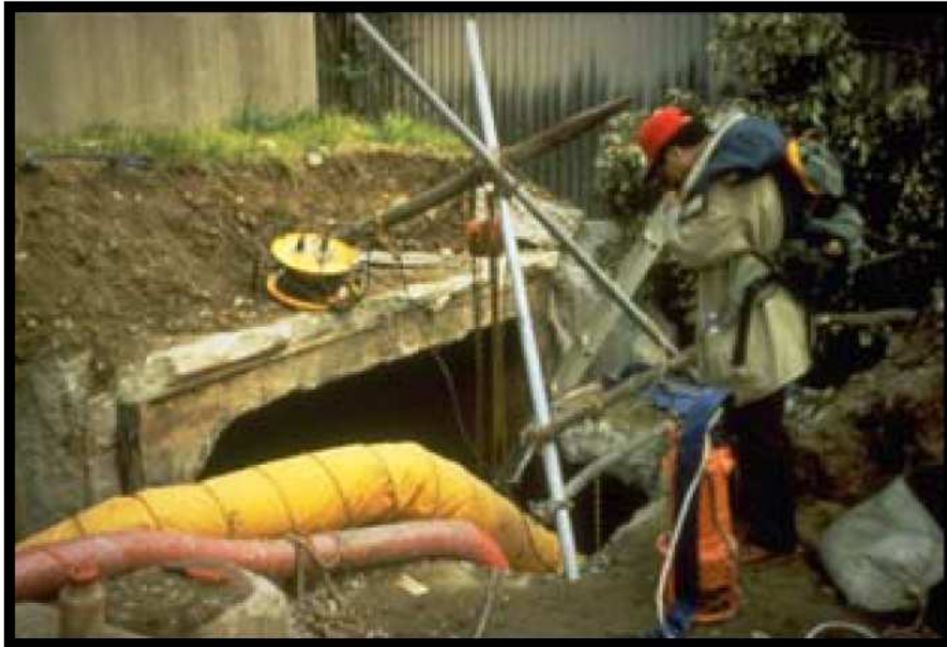
Example of main sewage treatment conduit rupture in the 1995 Kobe Earthquake Source – Kobe Geotechnical Collection, Earthquake Engineering Research Center, Univ. of California, Berkeley
