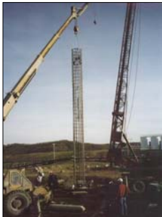
Once the Cage With Attached O-cell is Carefully Lifted, it is Installed into the Shaft Excavation
