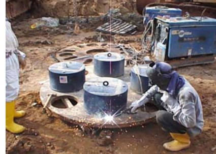
Multi-cell assembly - attaching O-cells to bottom plate
