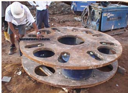
Multi-cell assembly - attaching top plate
