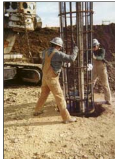
Once the Cage With Attached O-cell is Carefully Lifted, it is Installed into the Shaft Excavation
